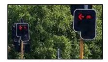
Figure 28: Cycleway signals with red turn arrow
