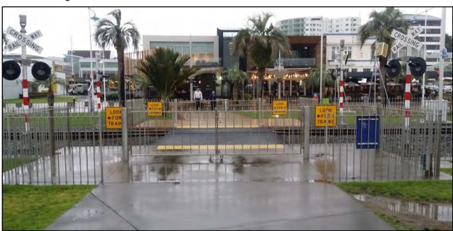
Figure 53: A double maze layout provides increased capacity at busy crossings – the design shown also provides an access gate for rail service vehicles (CBD, Tauranga)
