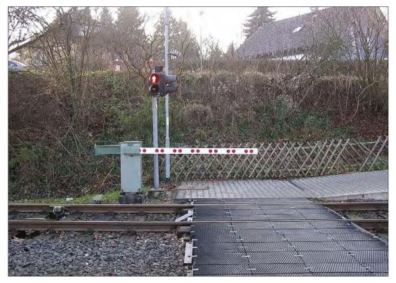
Figure 31: Example of pedestrian signals used with a barrier (Germany) (Wikimedia Commons)
