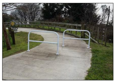
Figure 47: Example of alternating staples (may require side-fencing to avoid bypassing)
