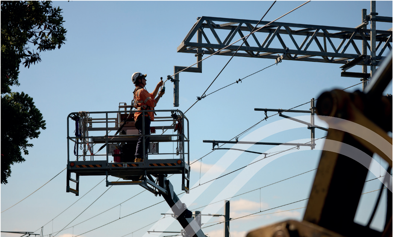
KiwiRail is renewing electrical overhead infrastructure for the future
