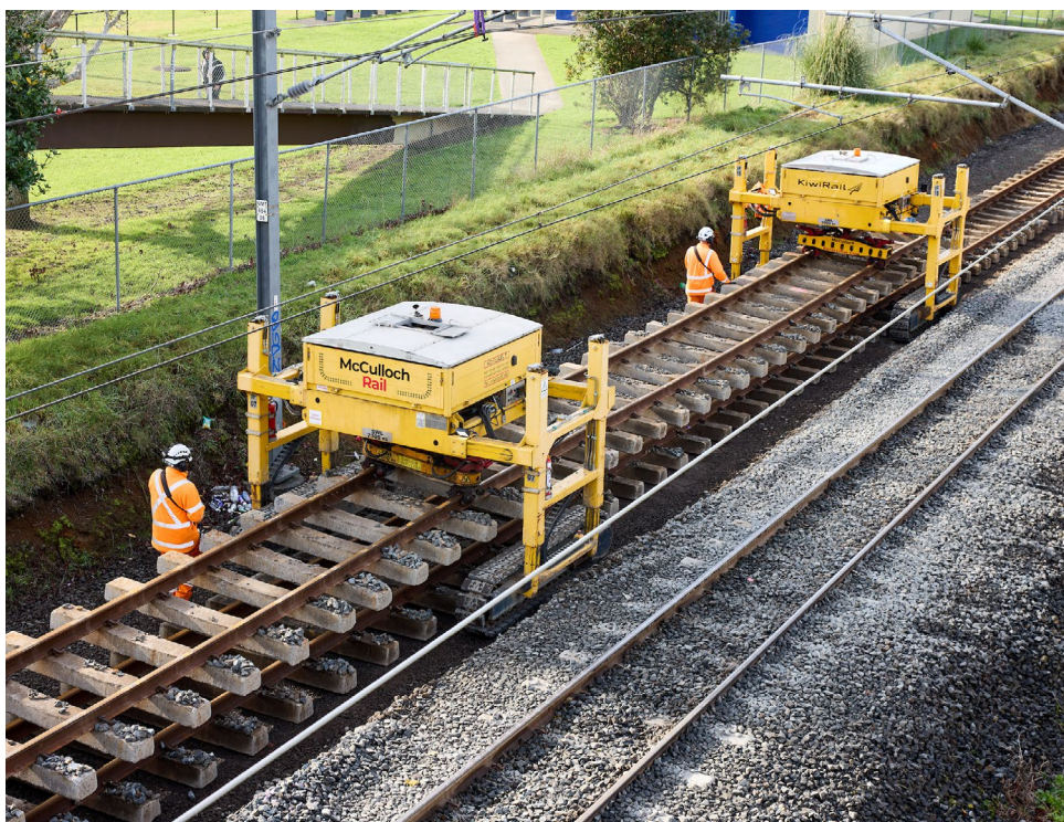
Panel Lifters in use in Homai. These specialist machines significantly reduce the time it takes to lift long sections of track when teams are upgrading foundations under the rails.
