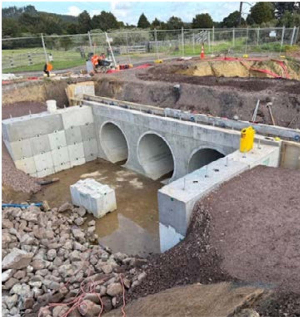
One of the barrel culverts being built
