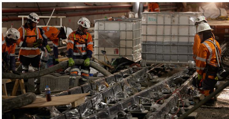
Pouring concrete under newly laid track at Britomart
