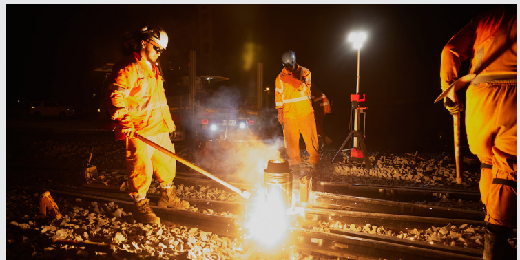
Night welding at Westfield Junction
