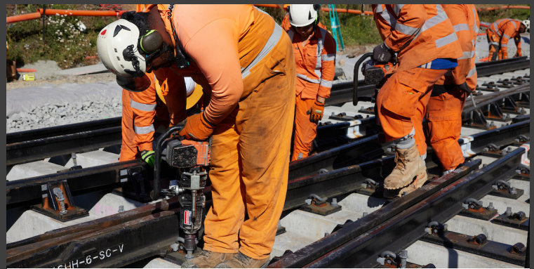
Helping to install the crossover at Pukekohe Station
