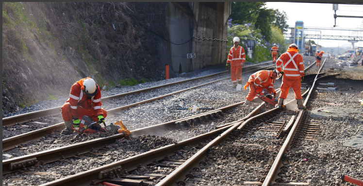
Removing tracks at the Pukekohe Station on Boxing Day
