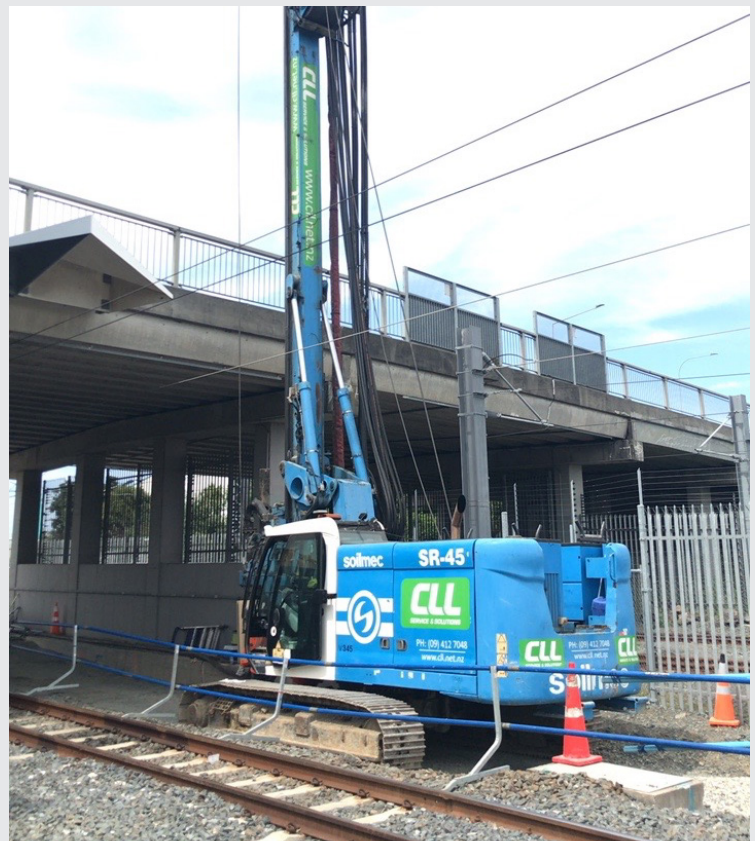
Piling works for the wall at the Wiri Station Rd bridge
