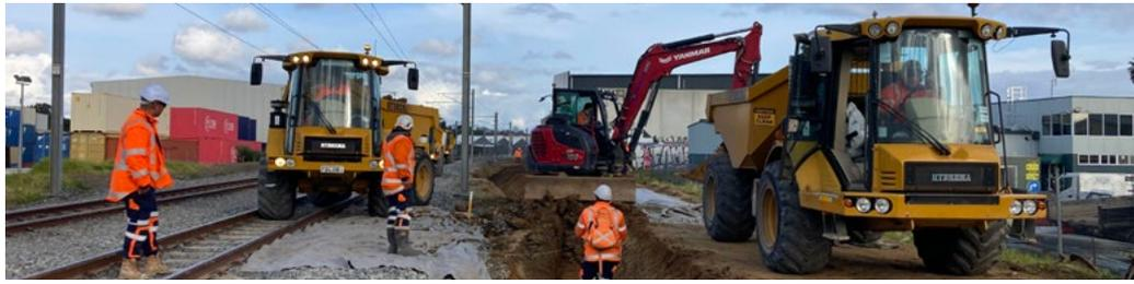
compacted rock foundation below the track) has been excavated and replaced
