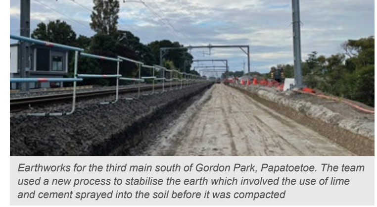
Earthworks for the third main south of Gordon Park, Papatoetoe. The team used a new process to stabilise the earth which involved the use of lime and cement sprayed into the soil before it was compacted
