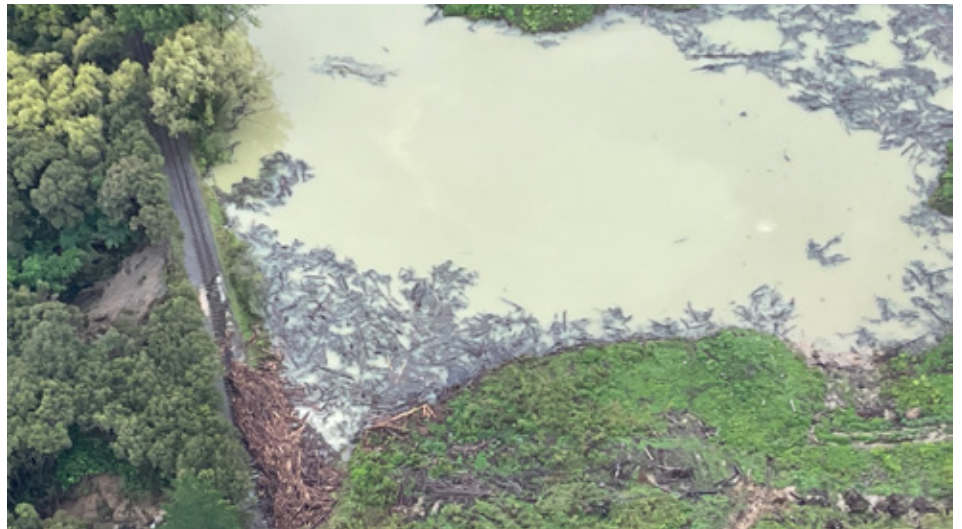
Example of a site that needs emergency works south of Waikoau between Napier and Wairoa
