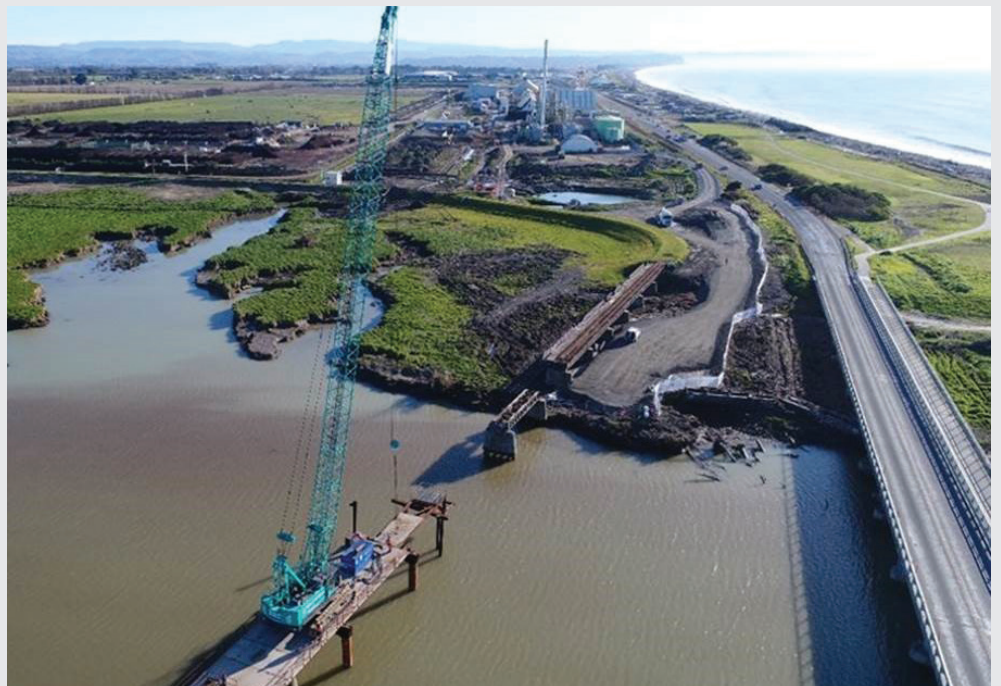
Good progress on temporary repairs to Bridge 217, Awatoto (south of Napier)
