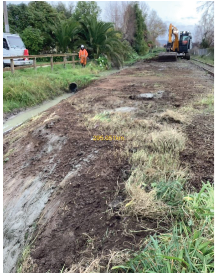
Clearing drains next to the track near Wairoa, to lessen flood risk over winter – before (left) and after (right)
