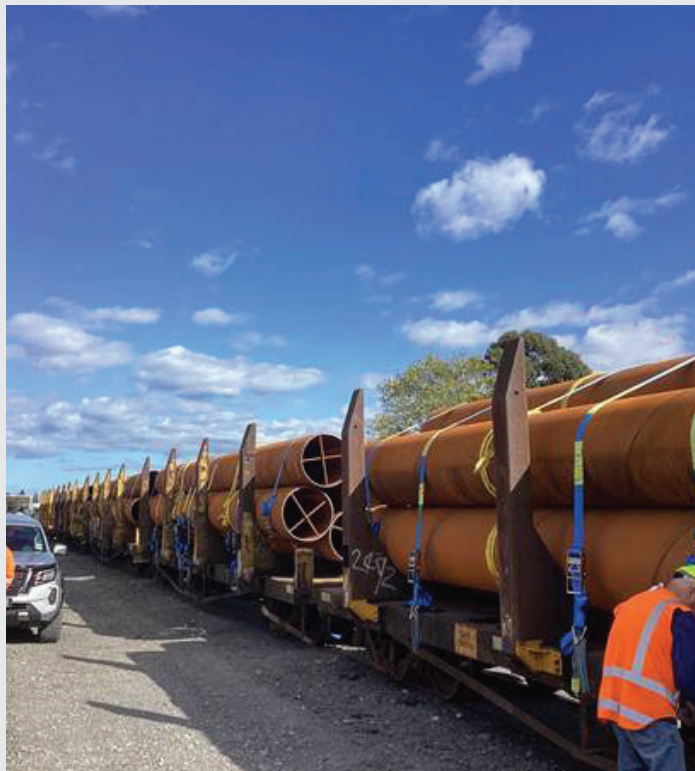
Train loads of steel casings, to act as temporary piers for the rebuild of Bridge 217, are being railed from Christchurch to Hastings.
