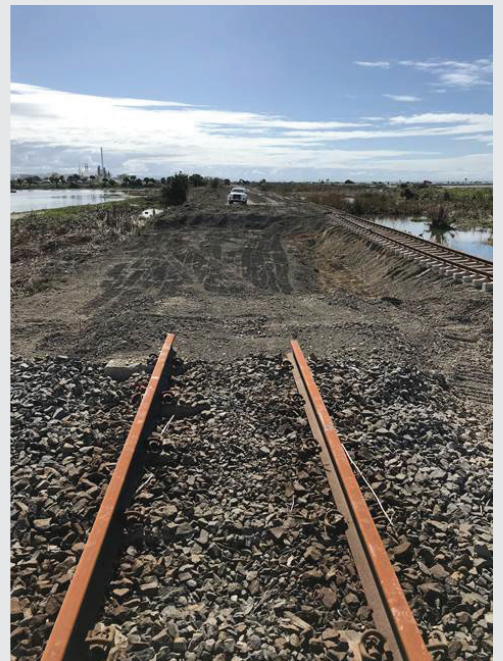
Example of damaged track being removed and the ground cleared around Awatoto – before (left) and after (right).
