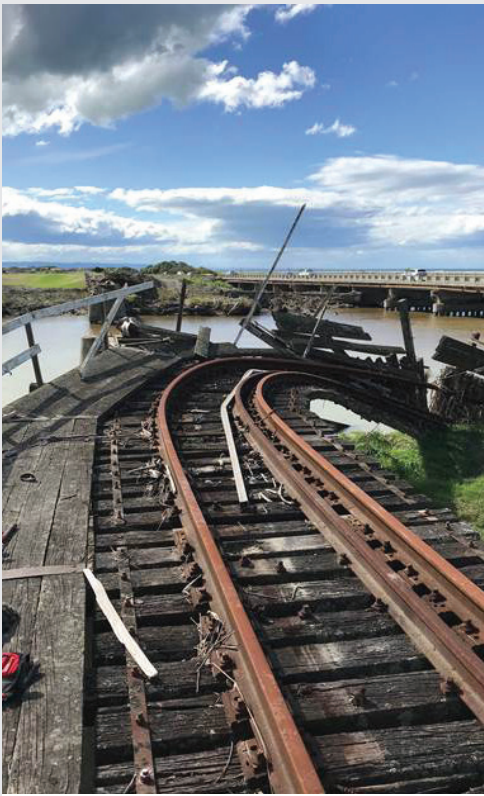
Rail removal on Bridge 217 – before (left) and after (right) – ahead of temporary repairs beginning.
