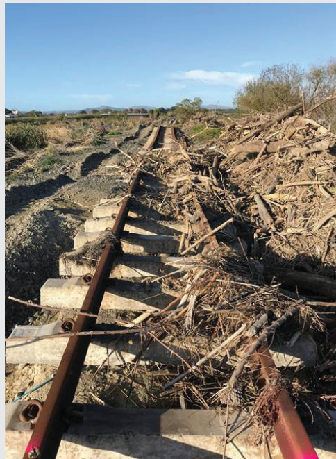
Example of damaged track being removed and the ground cleared around Awatoto – before (left) and after (right).
