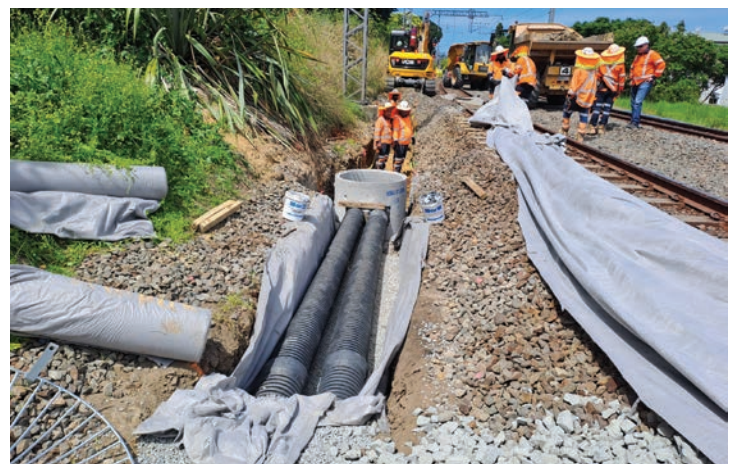
These pictures show old ballast and formation being excavated, and new drainage (subsoil pipes) being laid on the Western Line over Christmas
