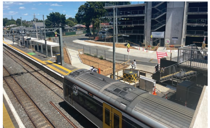
Works underway at Middlemore Station
