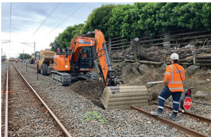
These pictures show old ballast and formation being excavated, and new drainage (subsoil pipes) being laid on the Western Line over Christmas
