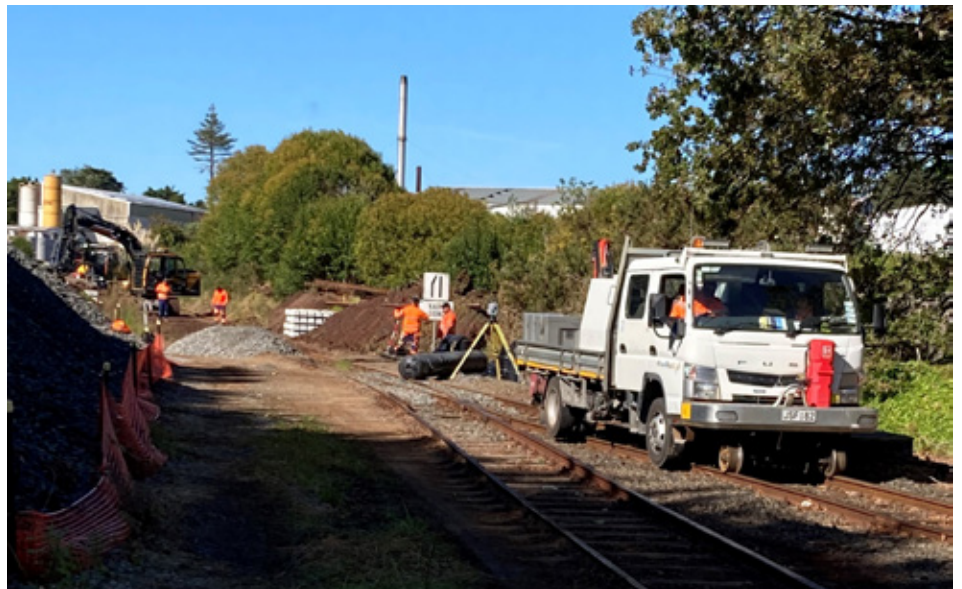
Northland - work getting underway to upgrade the rail line near Kauri
