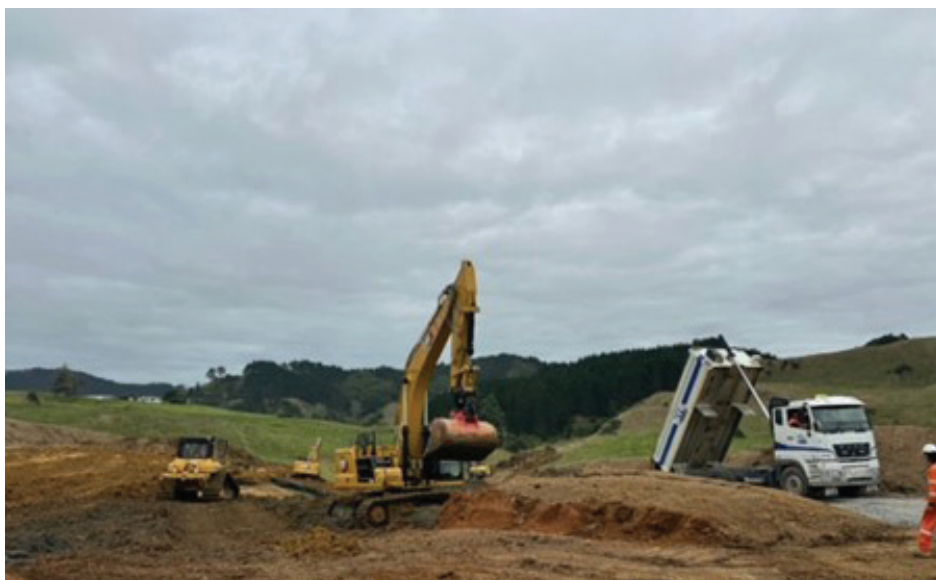
An example of a remediated site near Tahekeroa, where a slip prone hillside was excavated and an engineered rock structure (left of picture) built.
