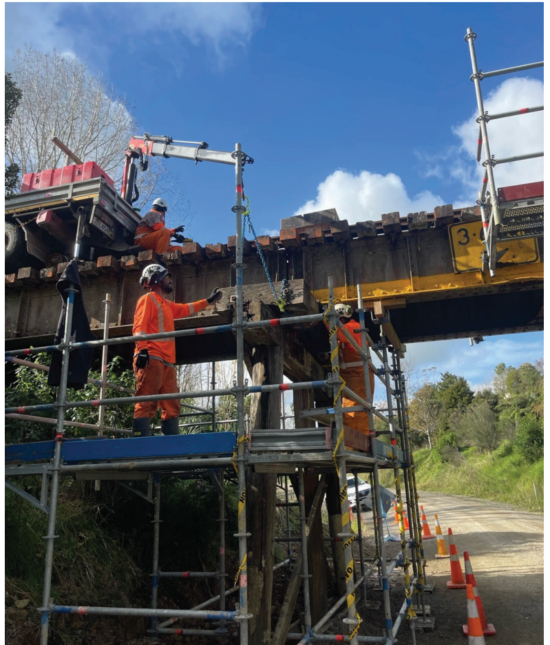
Work replacing a corbel on Bridge 140, Maungaturoto.
