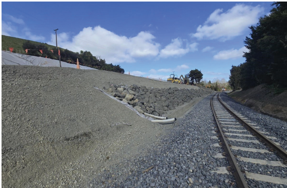
An example of a remediated site near Tahekeroa, where a slip prone hillside was excavated and an engineered rock structure (left of picture) built.
