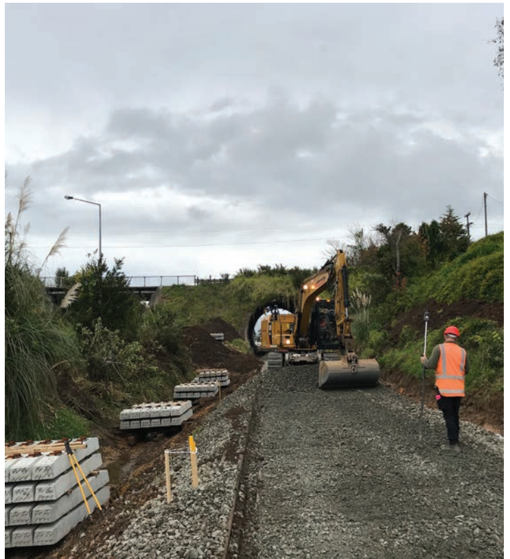
Track renewal and drainage work at Bridge 182 underpass
