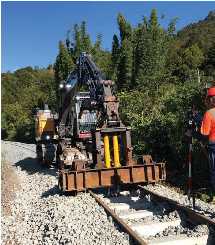
Lifting and alignment of track at Kauri.
