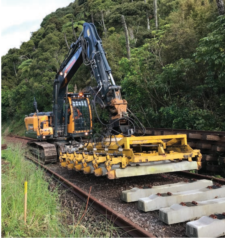
Installing concrete sleepers with sleeper laying frame at Kauri
