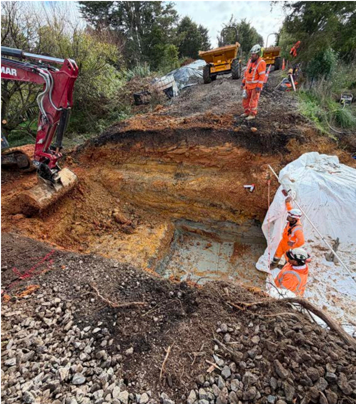
Installing a new culvert south of Wellsford, to protect the corridor from storm water flows.
