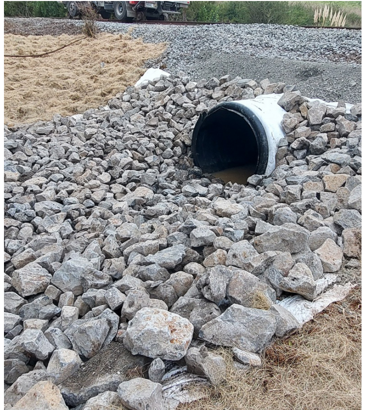
Installing a new culvert south of Wellsford, to protect the corridor from storm water flows.
