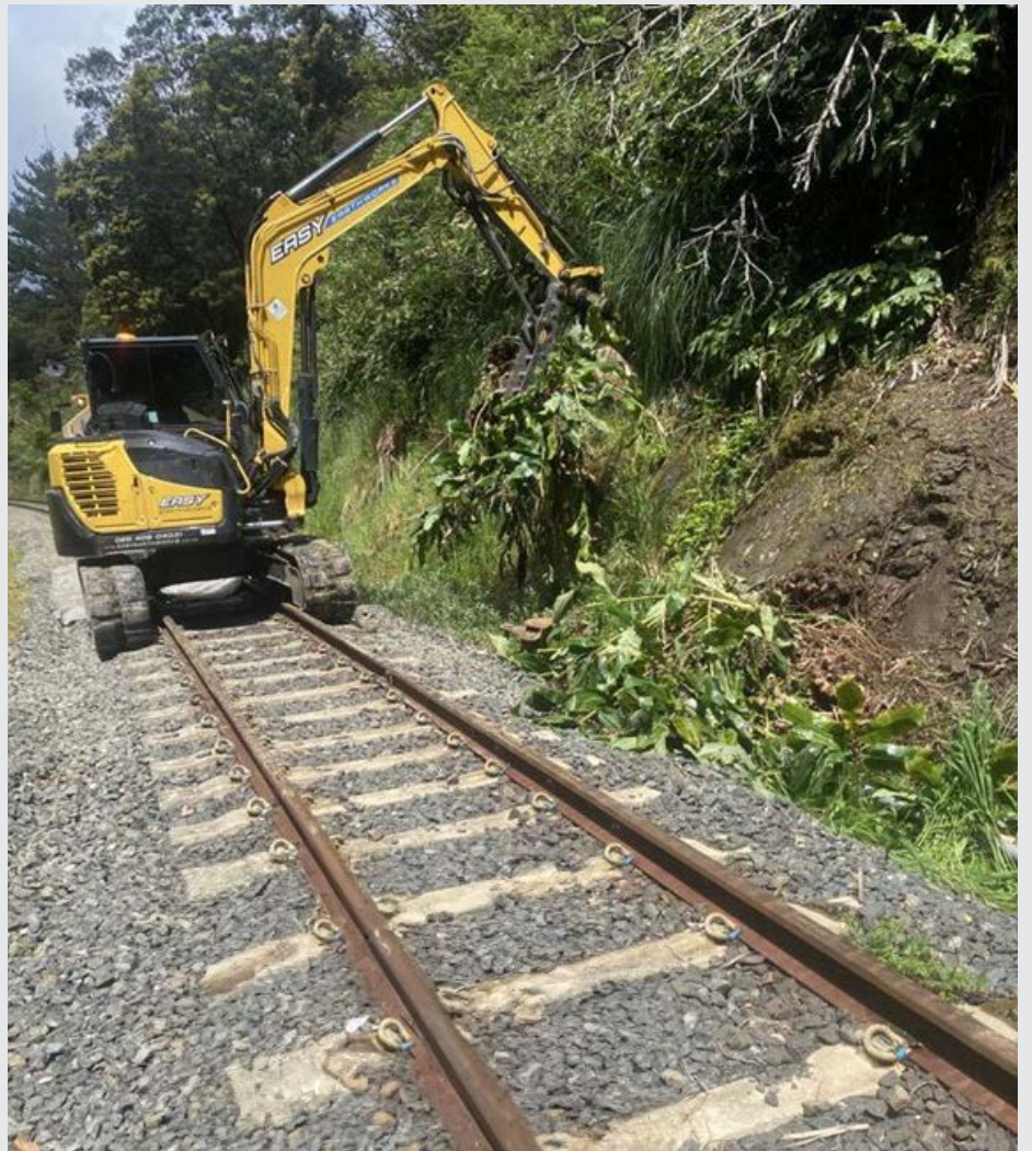
Clearing a small slip just south of Tunnel 1.
