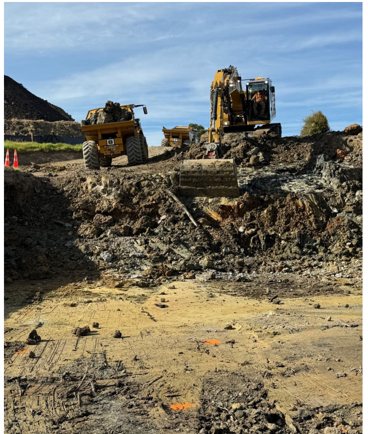
An example of Northland's slip prone geology. The excavation north of Waitira is where a gentle hillside slumped under the rail line. The track and ballast can be seen in the top left corner of the picture. This area will be rebuilt with sturdy material and improved drainage.
