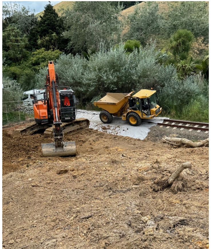
Work has begun clearing a slumped hillside above the tracks south of Mareretu. Drains will be installed in the slope to help stop more material coming down towards the tracks.
