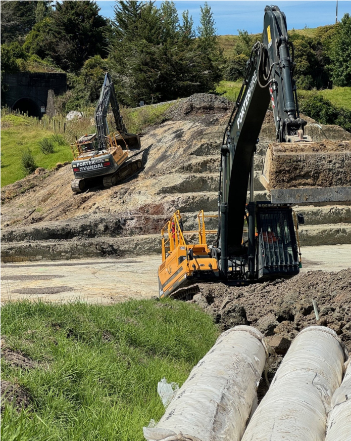
A massive slip below the rail line north of Ranganui, where a 100 metre length of embankment failed. About 21,000 cubic metres of unsuitable, saturated material, eight metres deep had to be excavated. The grey material on top of the “pyramid” is the ballast that the rail line sits in. The terraces cut into the earth will help tie the existing embankment into the new material which will be laid.
