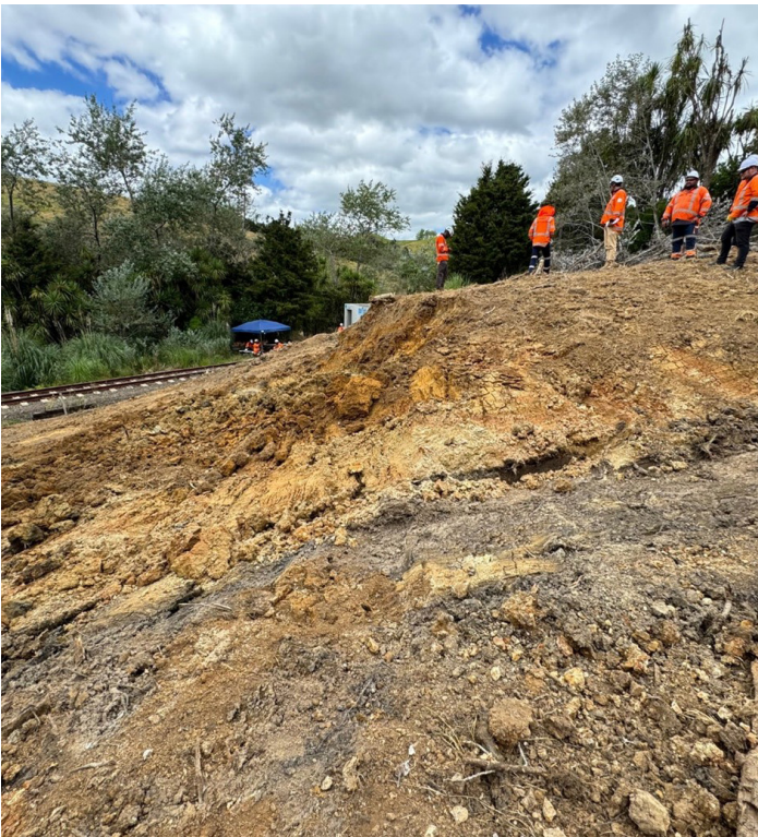
Work has begun clearing a slumped hillside above the tracks south of Mareretu. Drains will be installed in the slope to help stop more material coming down towards the tracks.
