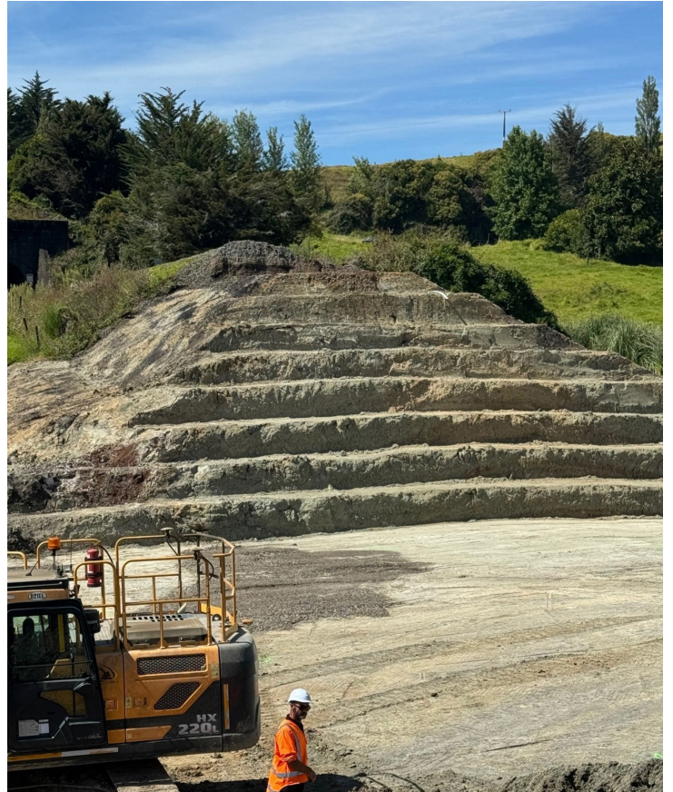
A massive slip below the rail line north of Ranganui, where a 100 metre length of embankment failed. About 21,000 cubic metres of unsuitable, saturated material, eight metres deep had to be excavated. The grey material on top of the “pyramid” is the ballast that the rail line sits in. The terraces cut into the earth will help tie the existing embankment into the new material which will be laid.
