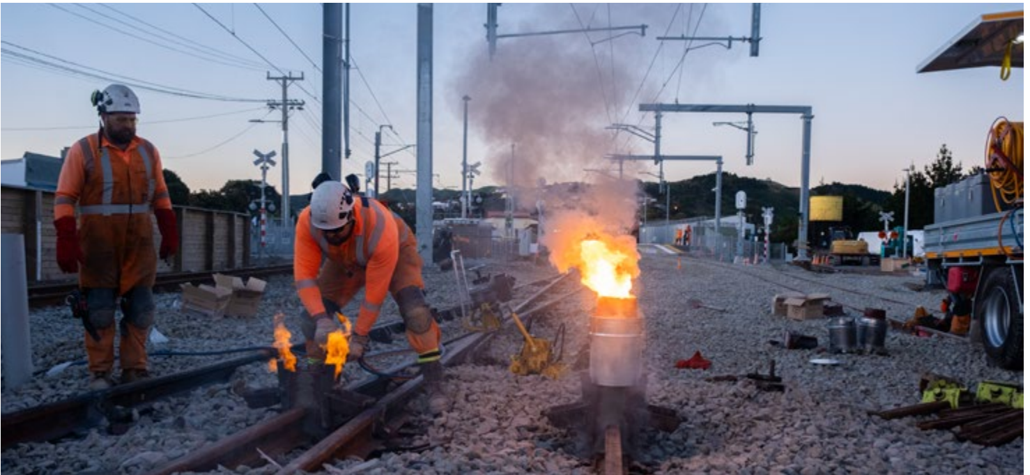
Welding sections of rail together at Plimmerton during the Christmas break
