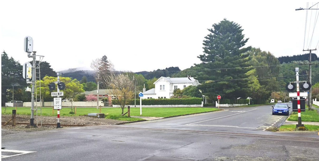
FIGURE 16 A TYPICAL LEVEL CROSSING IN THE WAIRARAPA
