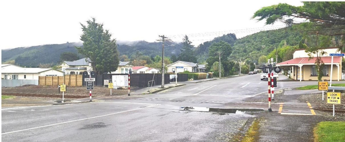
FIGURE 3 ACTIVE LEVEL CROSSING
