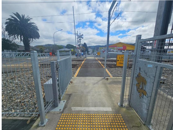
FIGURE 17 A PEDESTRIAN LEVEL CROSSING AT UPPER HUTT
