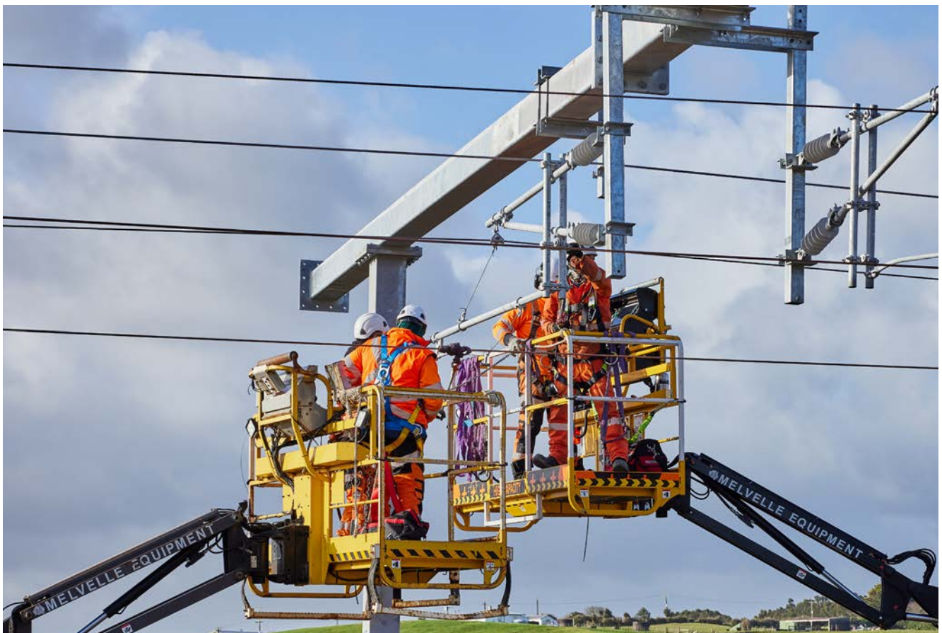
KiwiRail has been renewing its overhead traction systems, used to power commuter trains
