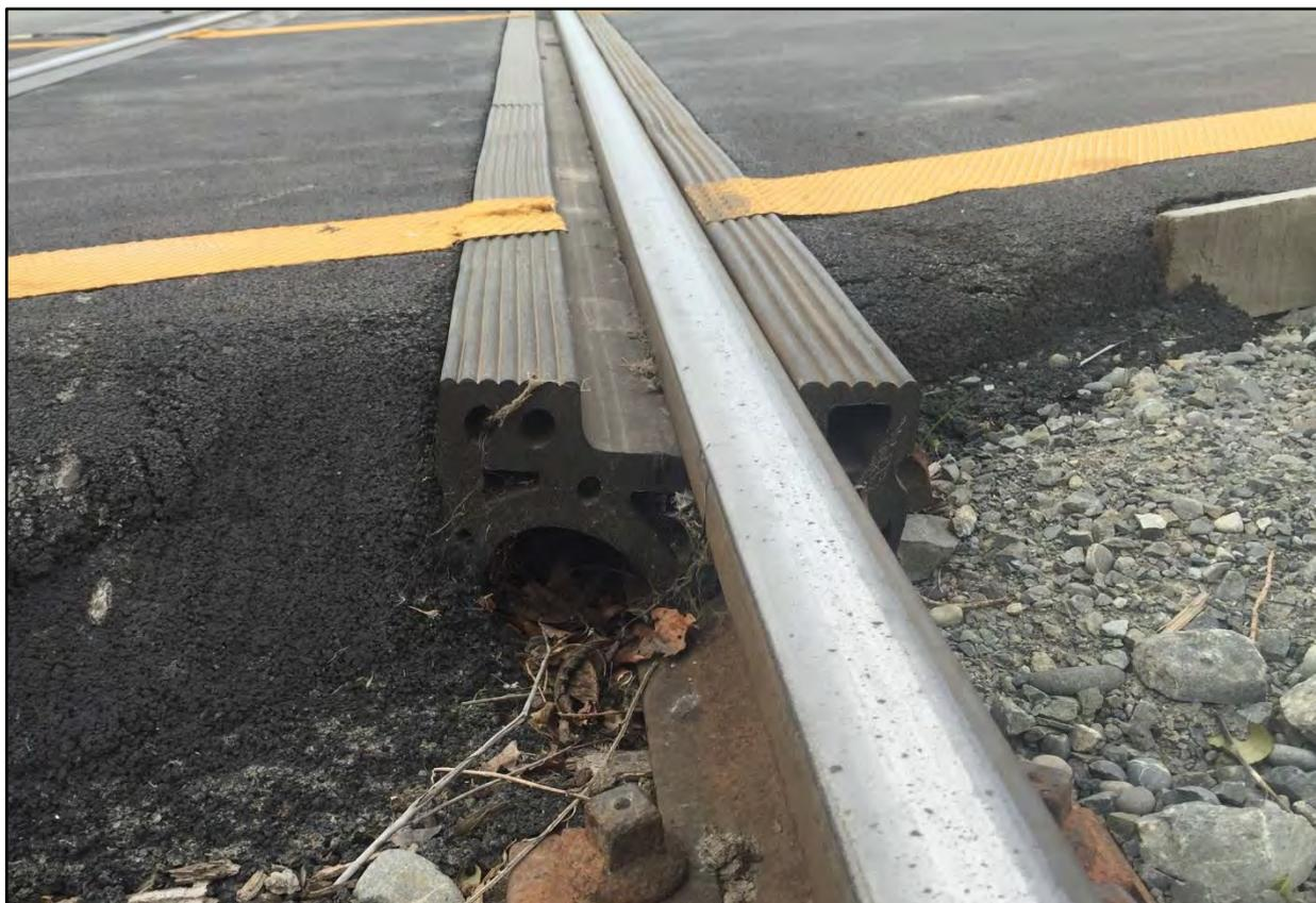
Figure 34: Eplex railseal used on asphalt railway level crossing (Kaiapoi)
