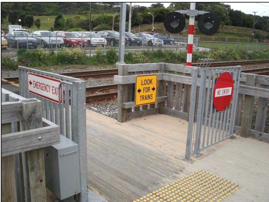
Figure 41: Automatic gate, normally open, with emergency exit to the right (Tawa, Wellington)
