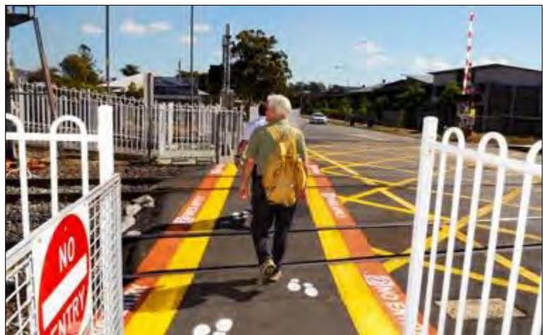
Figure 23: Example of Queensland Rail pedestrian marking trial
