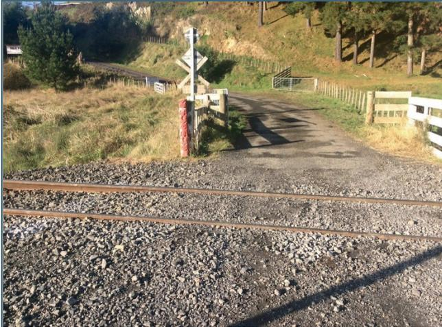
To ensure that adjoining owners have a level crossing that is best suited to their property type and usage KiwiRail now requires the use of 'timber panel', 'asphalt' or 'concrete slab' private level crossings surfaces which have lower maintenance requirements than gravel surfaces and help to prevent vehicles causing damage to the railway.
