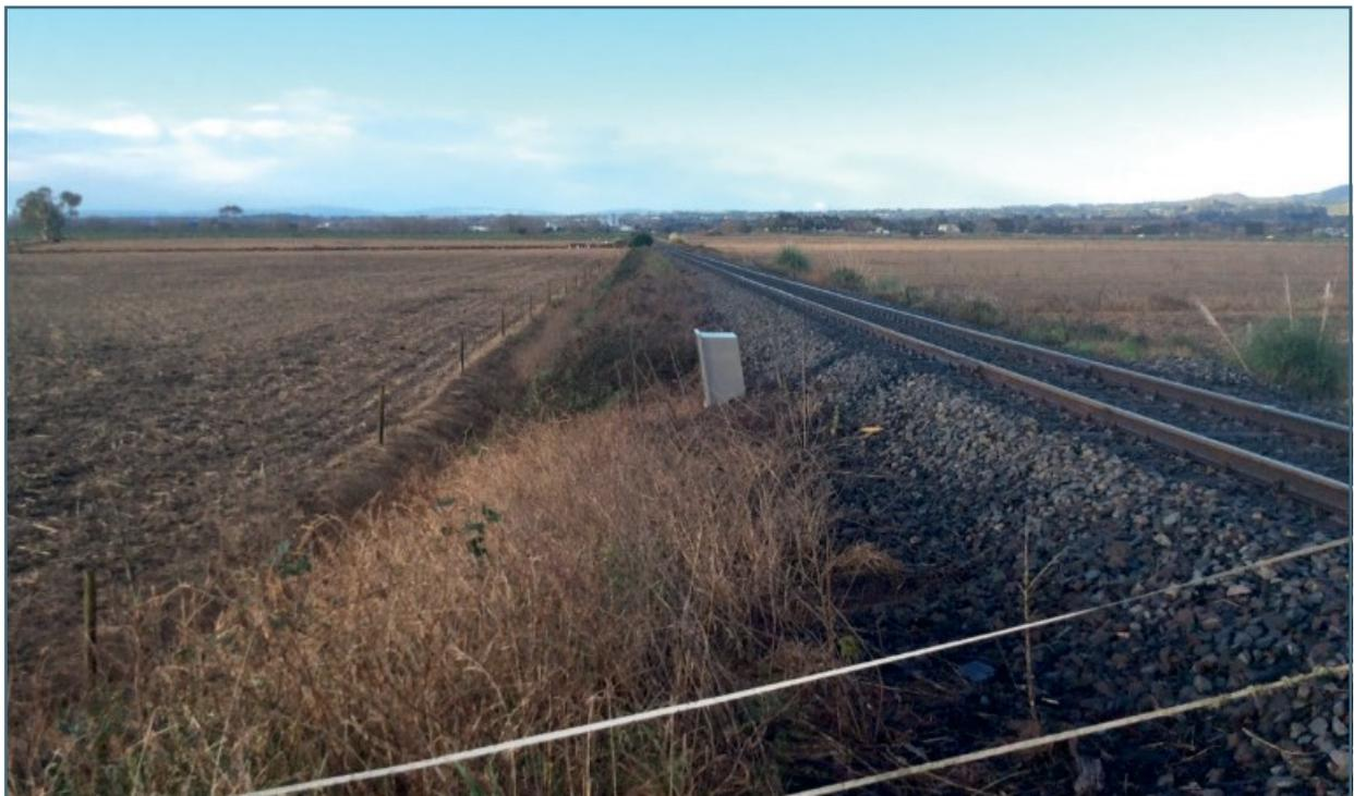
Unobstructed views up and down the rail corridor from 5 metres back from the railway track on either side of the level crossing
