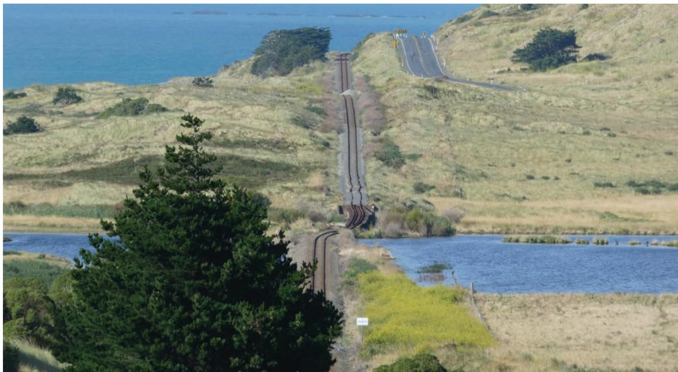
Bridge 129, Main North Line, moved approximately 0.6m horizontally and 2m vertically by the Kekerengu Fault during the November earthquake.
