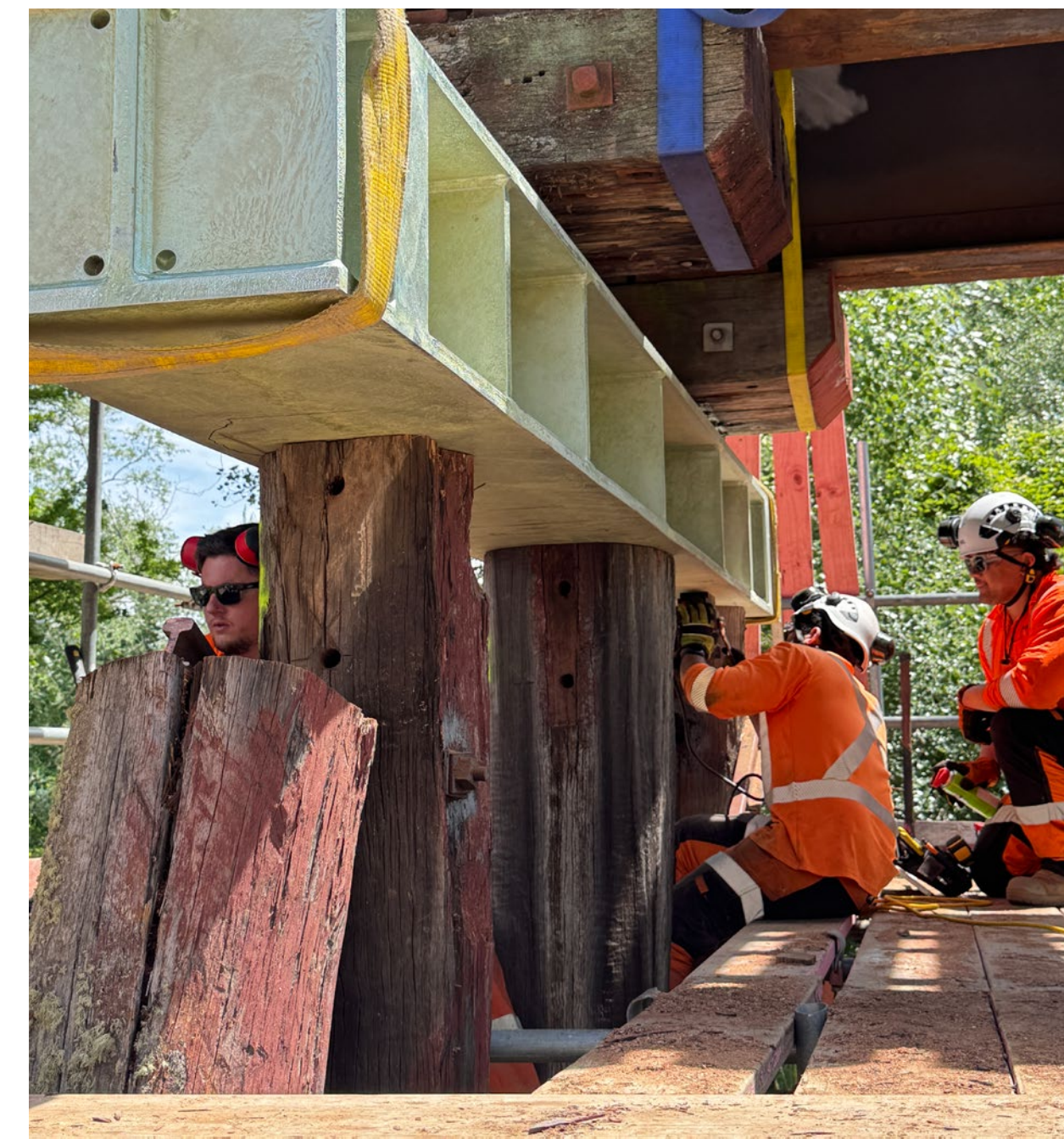
Bridge encasement extends the life of KiwiRail's bridge assets.
