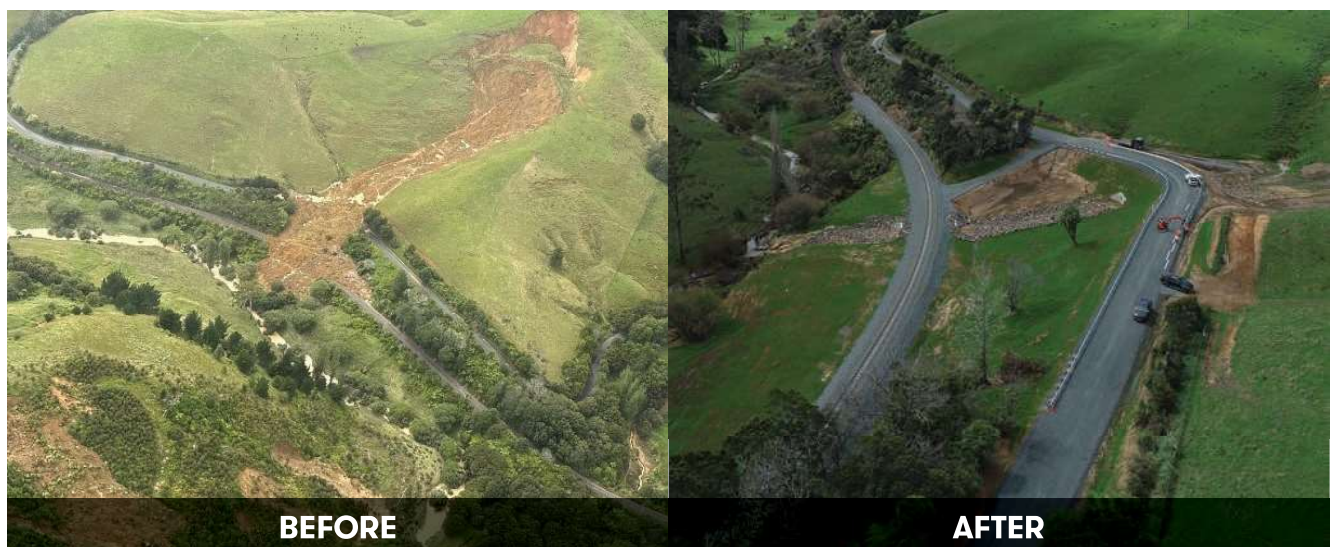
The slip at Tahekeroa blocked road and rail with 35,000 cubic metres of earth. KiwiRail’s repairs of the slip were completed in October 2023, with 95% of earth repurposed on site, saving thousands of truck trips and emissions and speeding up the programme by 10 weeks.
