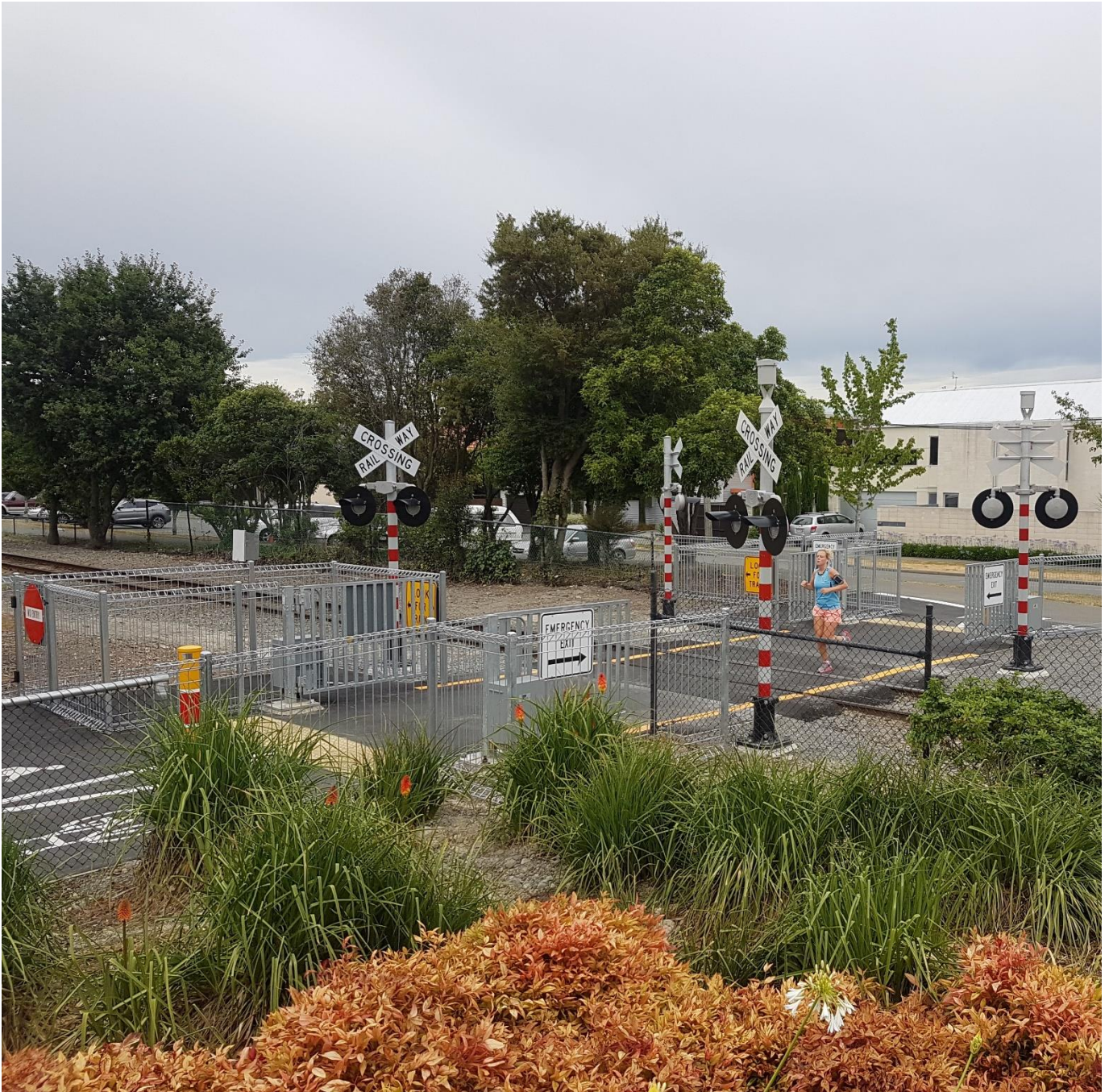
Image: Matai Street “saloon style” automatic gates shared path crossing (Christchurch, 2018)
