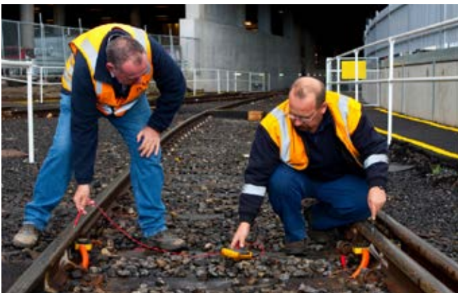
An outer flagman places detonators on a track
