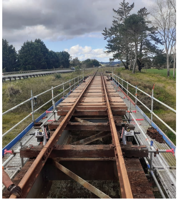
New sleepers being laid on Bridge 201
