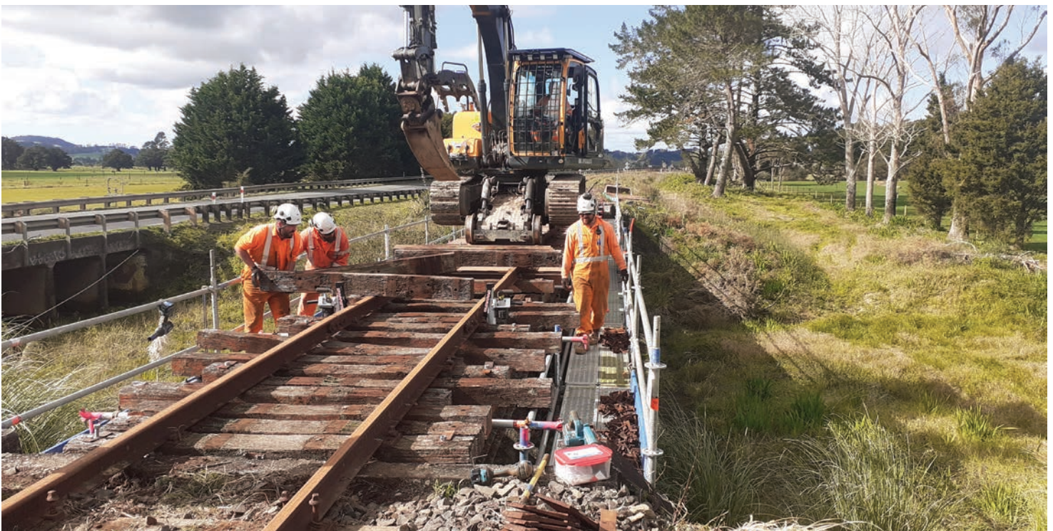
Removing old sleepers from Bridge 201
