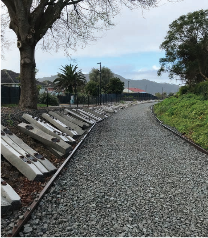
Ballast bed completed between Kamo Road and State Highway 1
