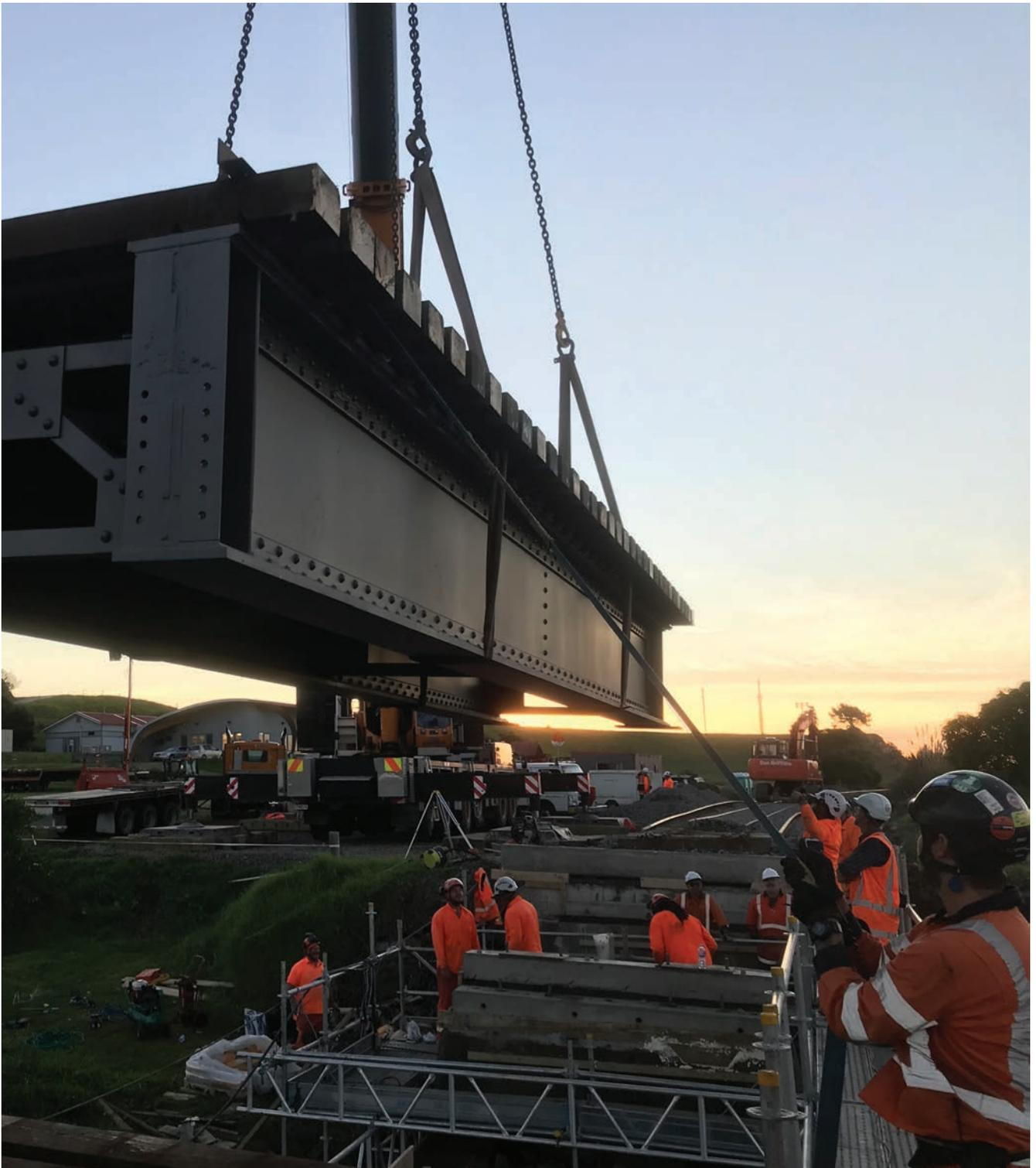
Refurbished steel span being lowered into place.
