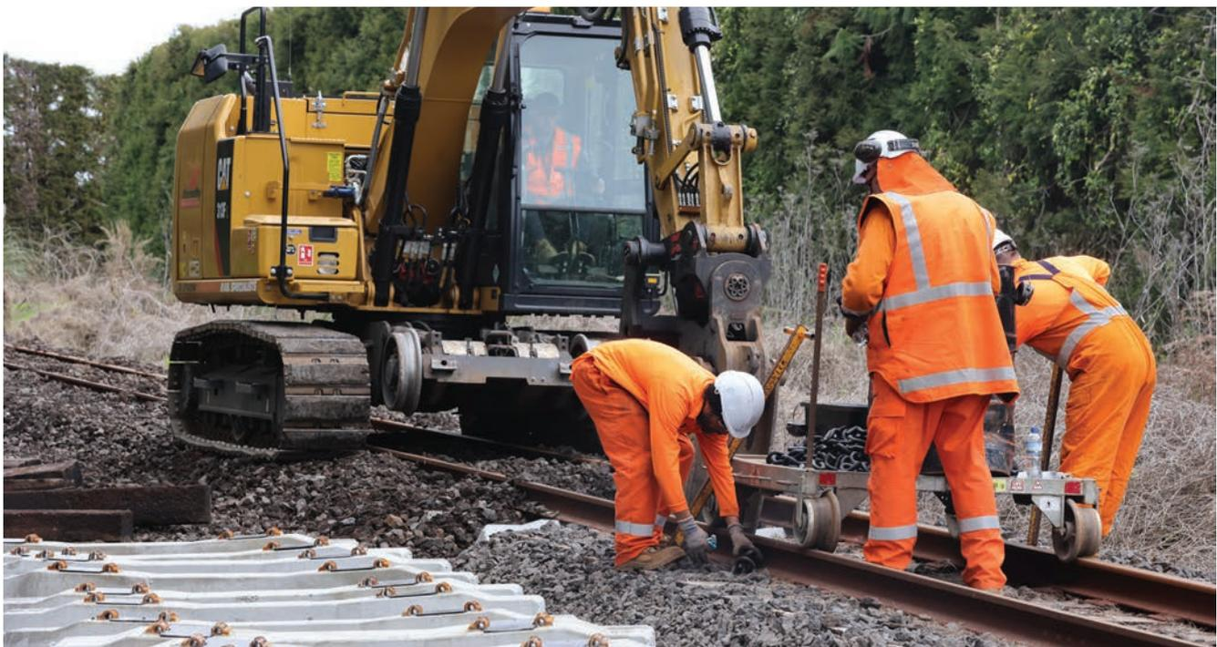
Timber sleepers being replaced with new higher strength and longer lasting concrete sleepers.
