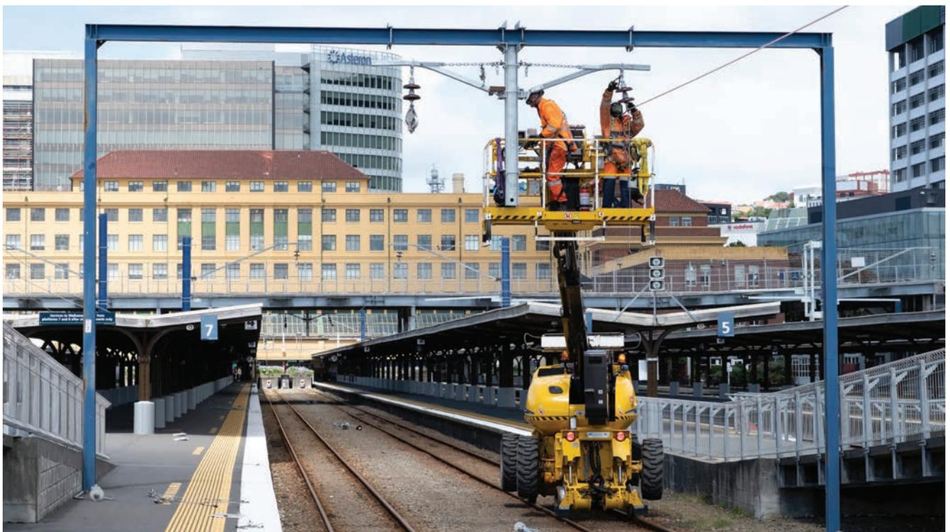
KiwiRail has been working to install modern tensioning systems in the Wellington metro area.
