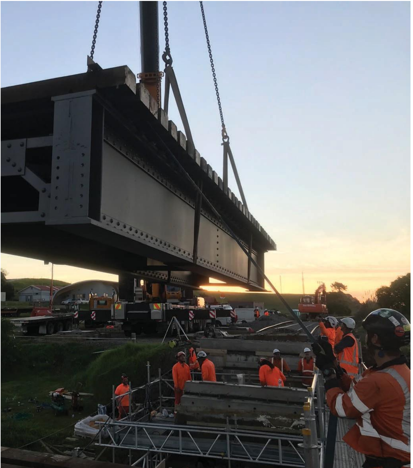
Refurbished steel span being lowered into place.
