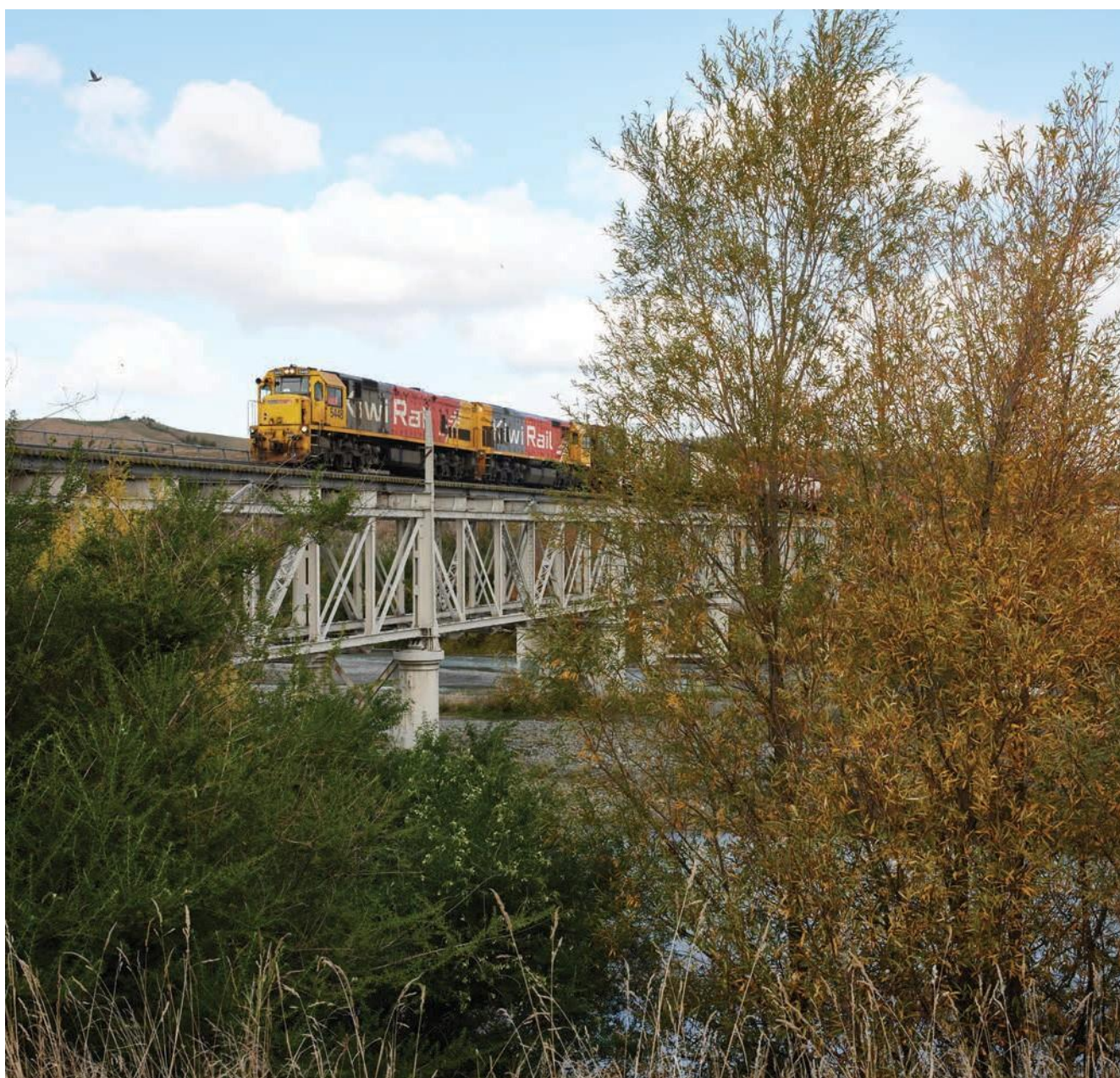
Crossing the Awatere River just north of Seddon.
